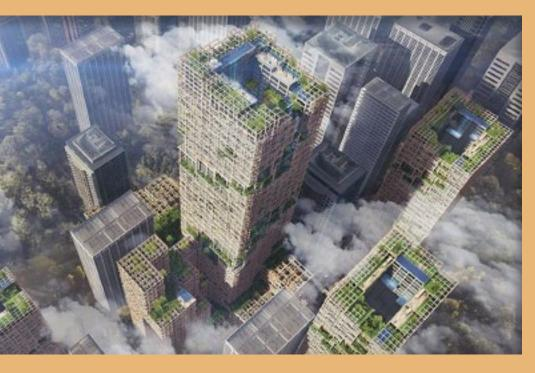
A Japanese company is set to build a skyscraper made of 90% wood in Tokyo, which will make it the world's tallest wooden skyscraper upon completion. The wooden high-rise, named "W350", will be a "braced tube structure" at 350 meters (1,150 ft) tall and 70 stories. To construct it, 180,000 cubic meters of wood will be combined with the other 10% of the building's makeup—steel.
